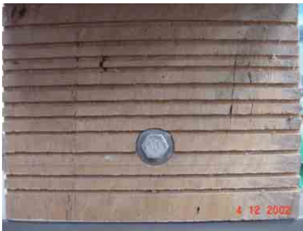
Landing pad with counter sunk coach screw head
